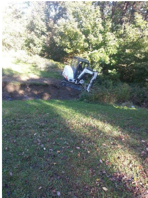
Leach field repair
