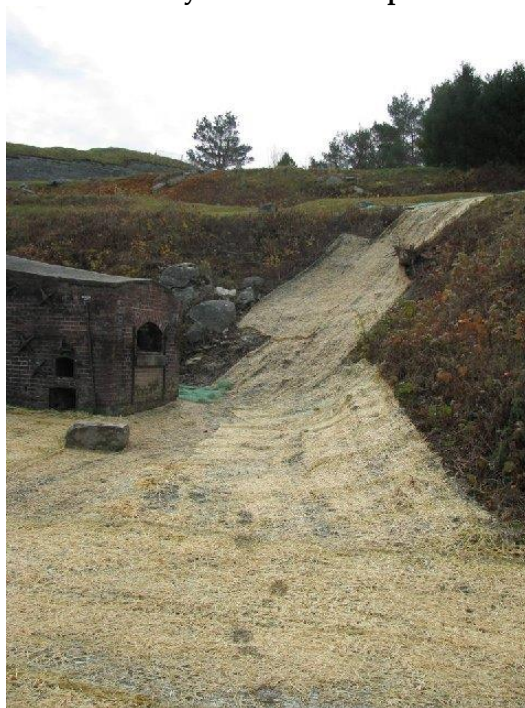
Battery B repair
